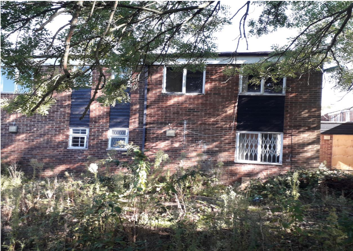
Rear elevation of application building
