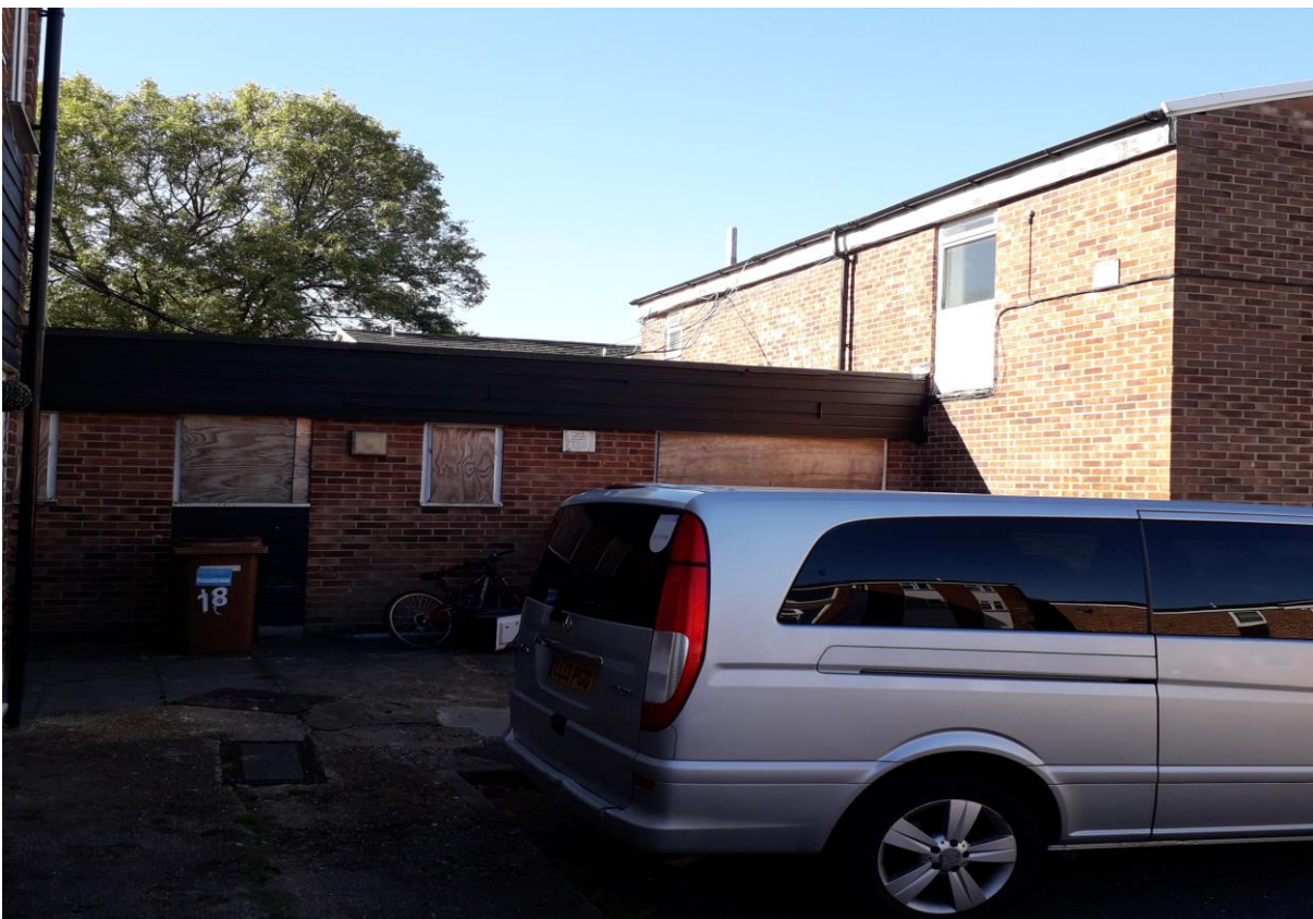
View of application building
